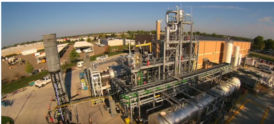
Figure 9 – Picture of a pyrolysis plant converting 25,000 tonnes of plastic per year
